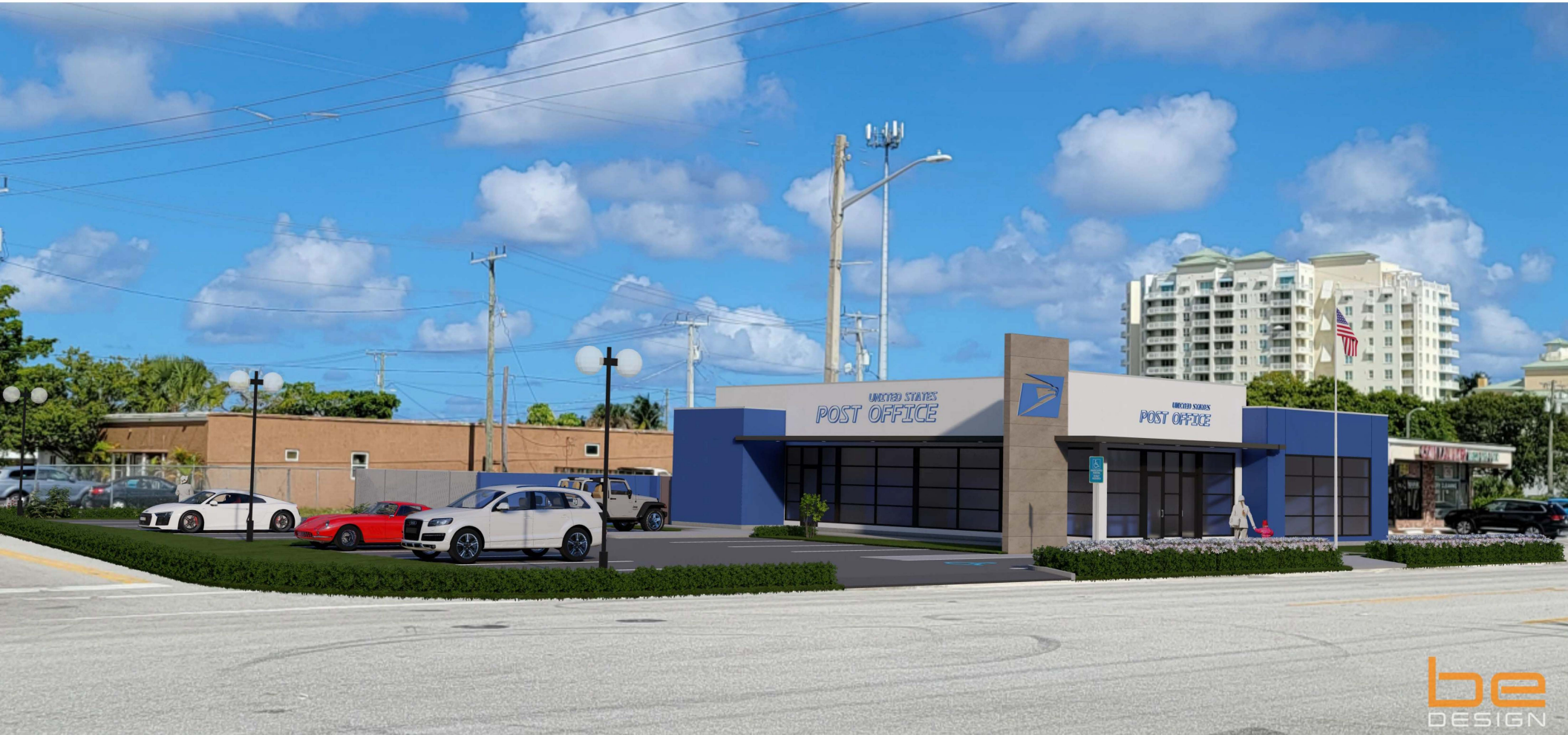
Main View from Southwest
